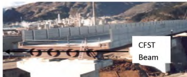
Fig.1. CFST beam in Bridge of Shinkansen –Japan [1]
